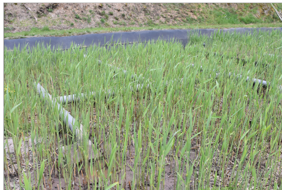
Figure 2.10: Reeds growing in the first stage of Montromant's VFTW
